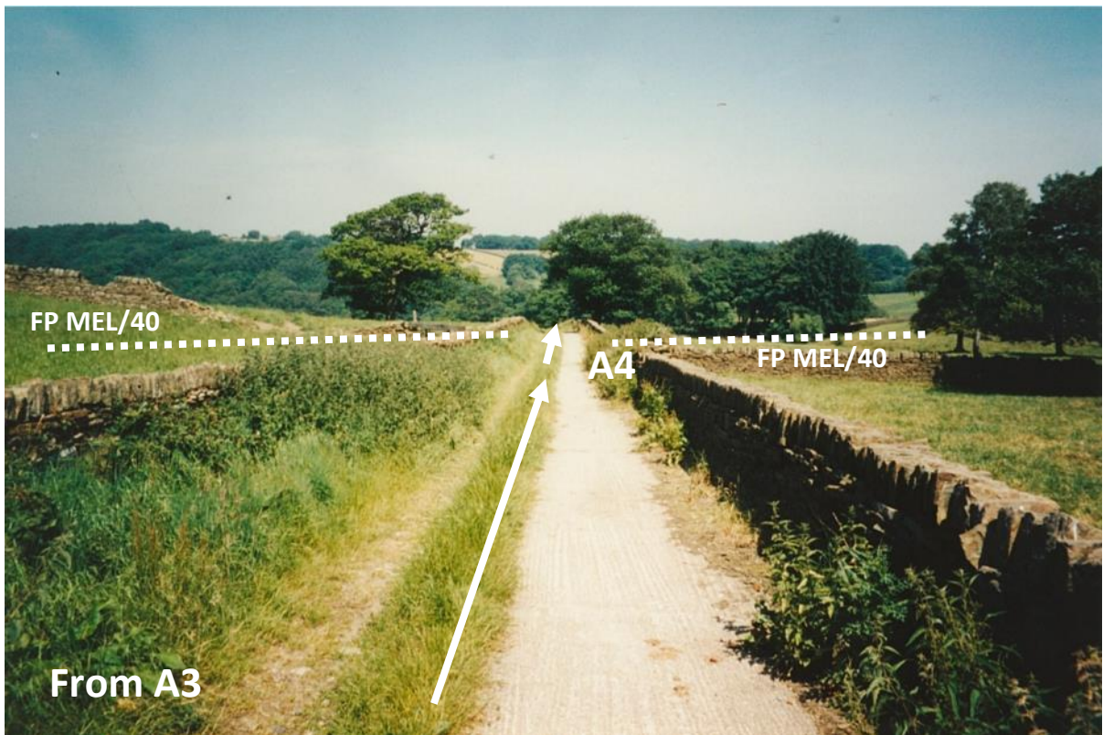
19. Meltham 70 south of point A4. The concrete surface appears only to cover part of the width, with a stone and grass surface alongside. Taken by Kirklees Council staff 1994 or 1995.
