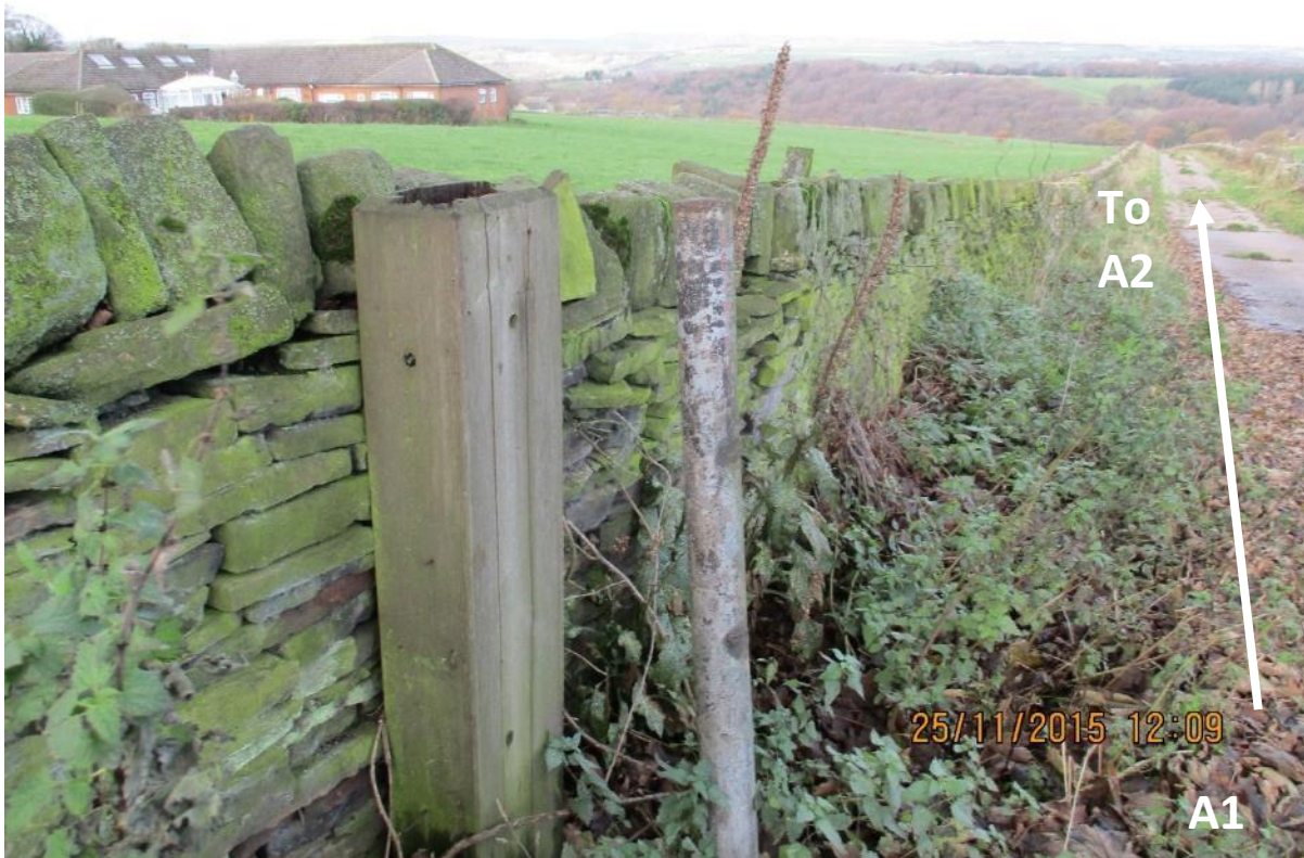
8. Wooden gatepost and metal pole on west side of Meltham 70 at point A1. 25 Nov 2015.
