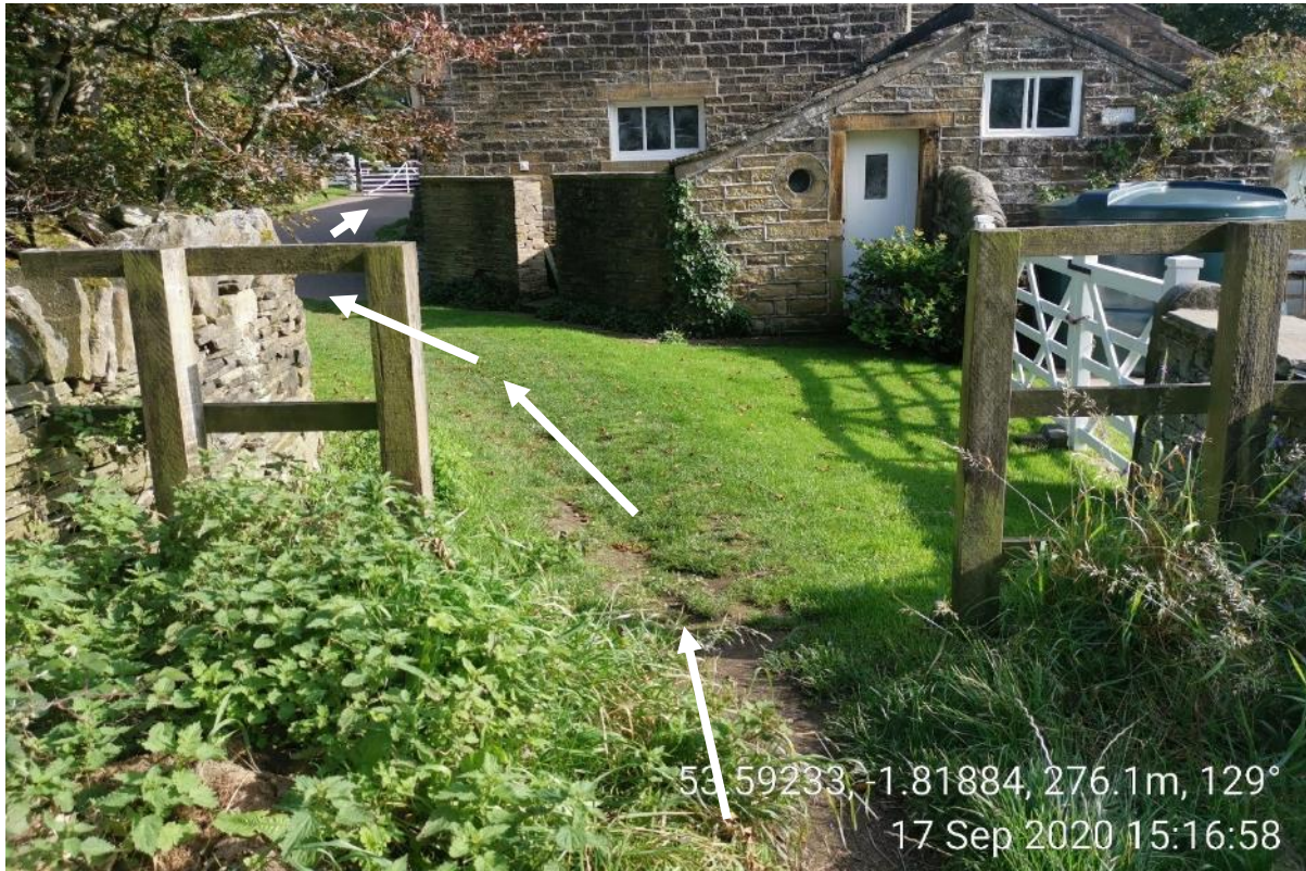
42. Barriers at Point C on Meltham 38 at Wood Nook House. 17 Sep 2020.
